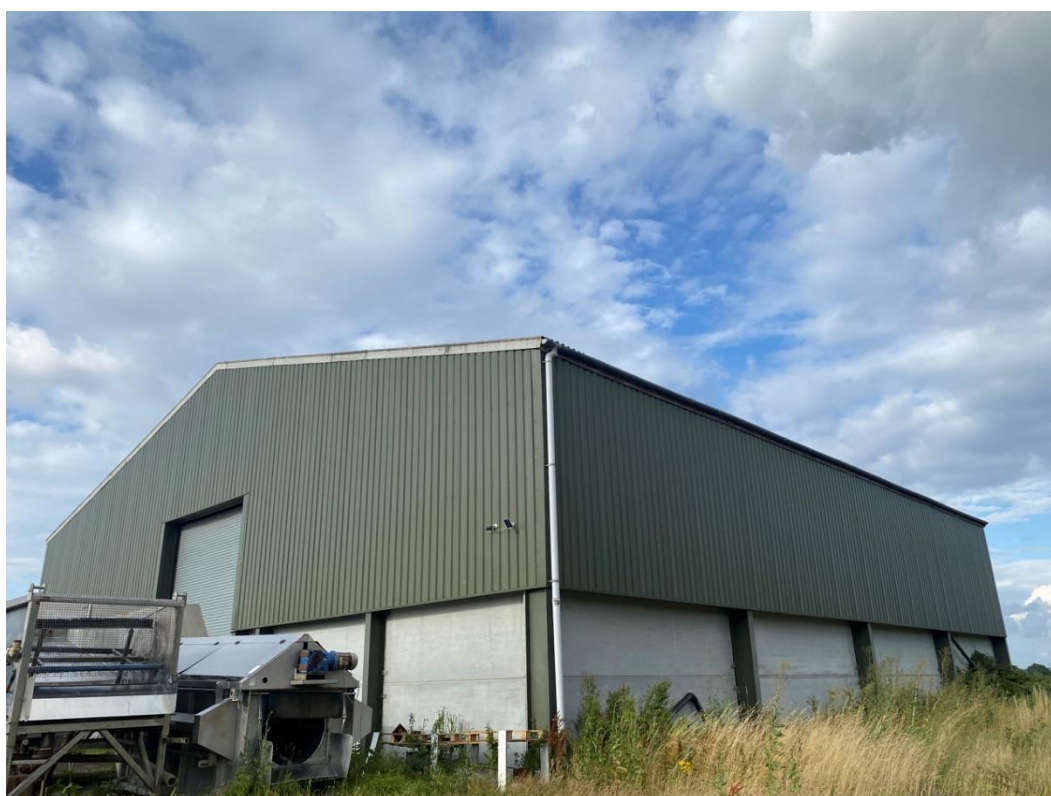
Figure 3-13: Existing Barn within Field NW08 of the Solar PV Site
